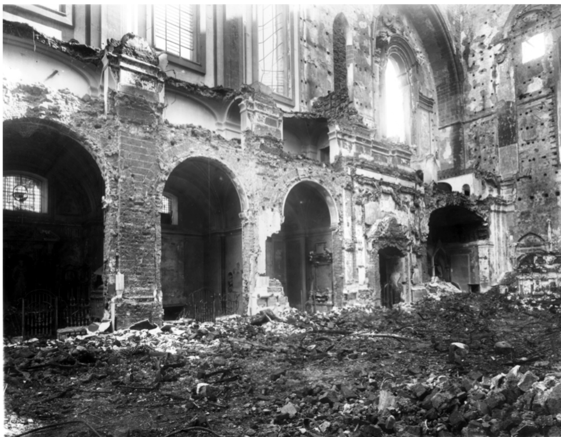
Figure 2 – The Basilica of Santa Chiara in the aftermath of August 4th, 1943 bombing (ASBAN, B2187)
