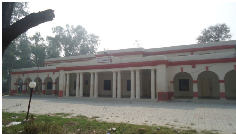
Figure 15 Dak Bungalow, Sheikhpura. Source: Photograph taken by the Author.
